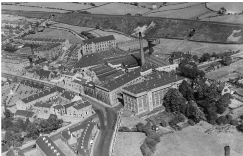
The main Clifton Mills at Bailiff Bridge from the air
